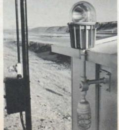
By the use of a reserve indication relay in series with the lamp filament, NP provides an approach aspect on the preceding signal when a lamp failure occurs. Power-off relays are provided to introduce approach lighting in the event the commercial power fails. The signals are then lighted from the reserve battery.
