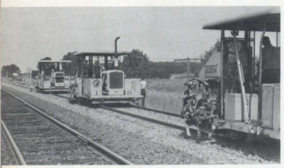
NORTHERN PACIFIC uses two conventional tampers (right) working in tandem with an automatic tamper at left. This technique increases production of surfacing gang.
