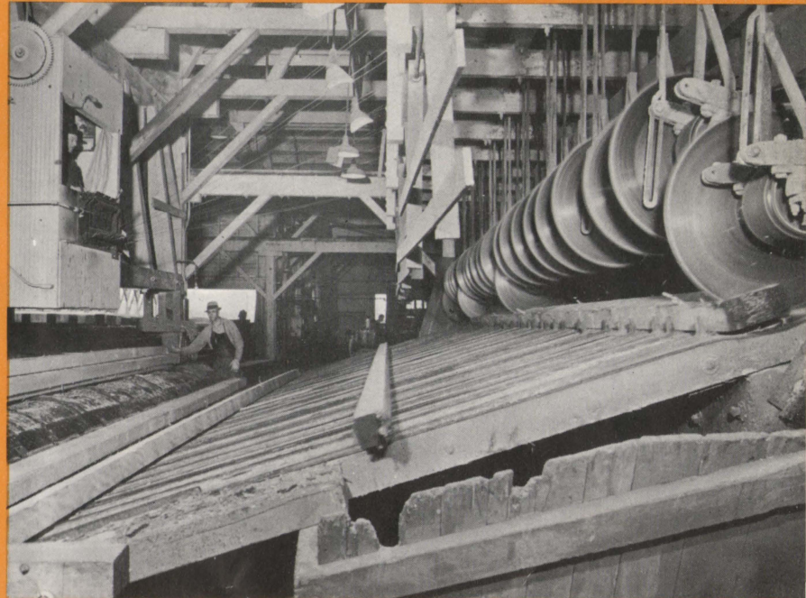
Trimmerman manipulates his 21 saws like an organist at the keyboard. He trims out defects in the lumber, and cuts to desired lengths. His decisions must be swift.
