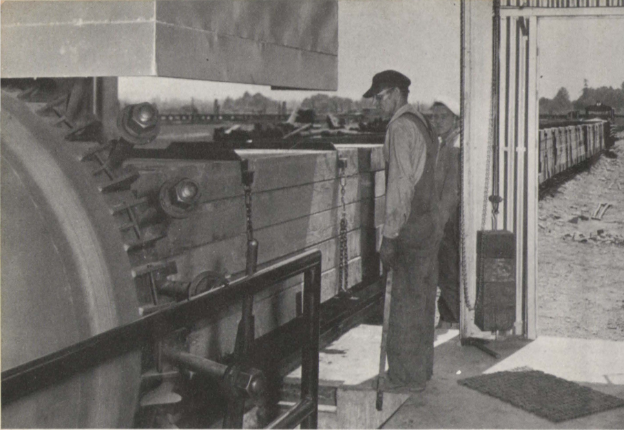
On Everett Lumber Division's millsite is a modern lumber treating plant, which chemically impregnates construction and railroad timbers for specific uses.
