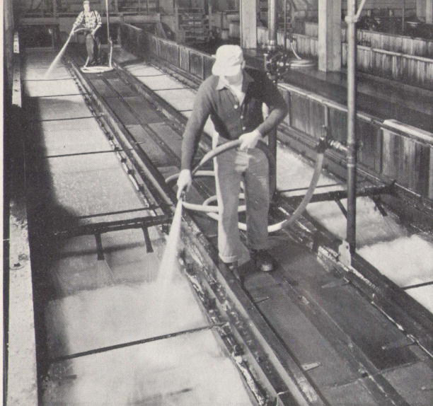
Unbleached pulp going over flat screens
