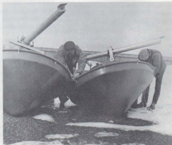
TWO PARABOLIC antennae are readied by workmen on building roof prior to being hoisted up and attached to tower.
