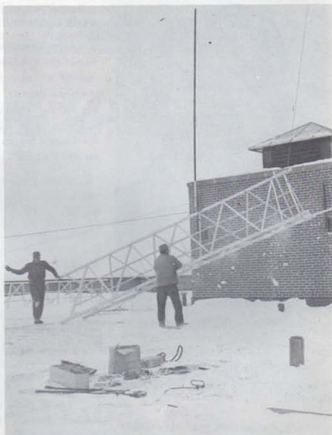
TOWER SECTION rises as workman signals power operator to lift steel framework to top of tower sections already in place. Lying in snow in foreground are tools and supplies for tower installation.
