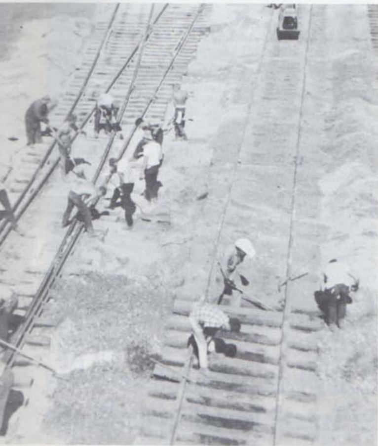
NP CONSTRUCTION crews at work in Missoula classification yard cleaning ballast from tracks.
