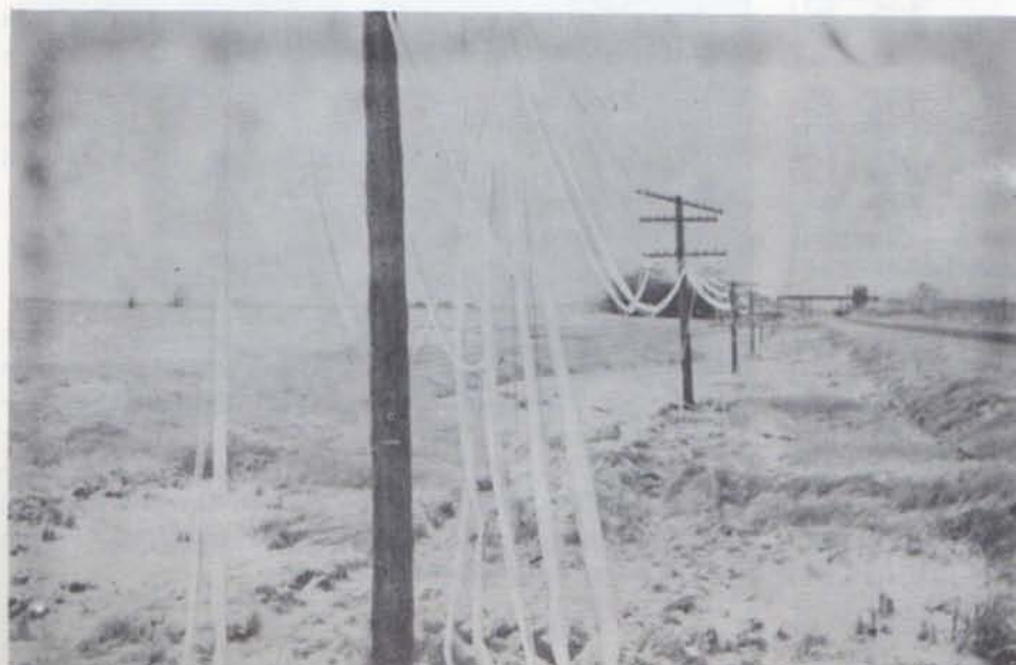
COMMUNICATIONS LINES, broken by the weight of ice encasing them, droop to the ground like giant strings of spaghetti. Twisted and broken wires were a common sight in the storm swept area.
