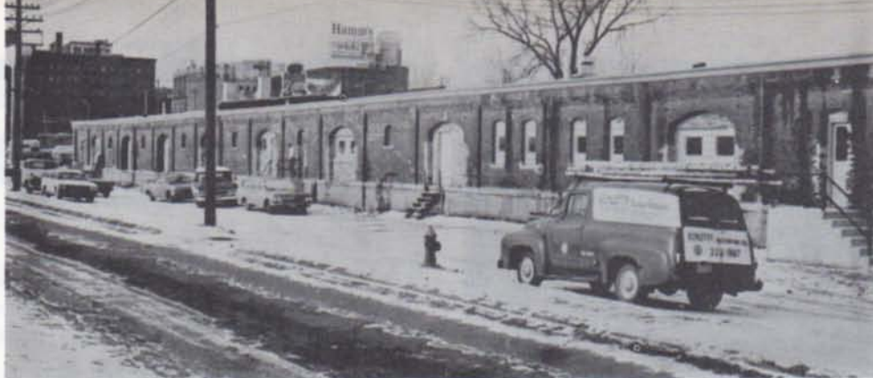
NORTHERN PACIFIC'S remodeled St. Paul freight office, located on Fourth Street, during the final stage of construction work. New windows and doors replace former steel openings on this street side. The building provides 24,000 sq. ft. of space, and houses 26 new rooms and offices divided among five company departments. At the left, a Lafayette bridge pier towers over the building's west end.
