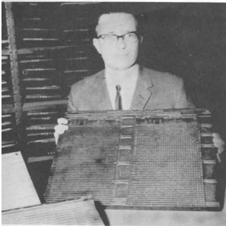
COPPER PLATES , like the one held here by J. F. Woodburn, buyer in the stationery section, are used to reproduce printed forms required by the Northern Pacific. Plates are stored on shelves in background. On table in front, lies a white zinc plate.
