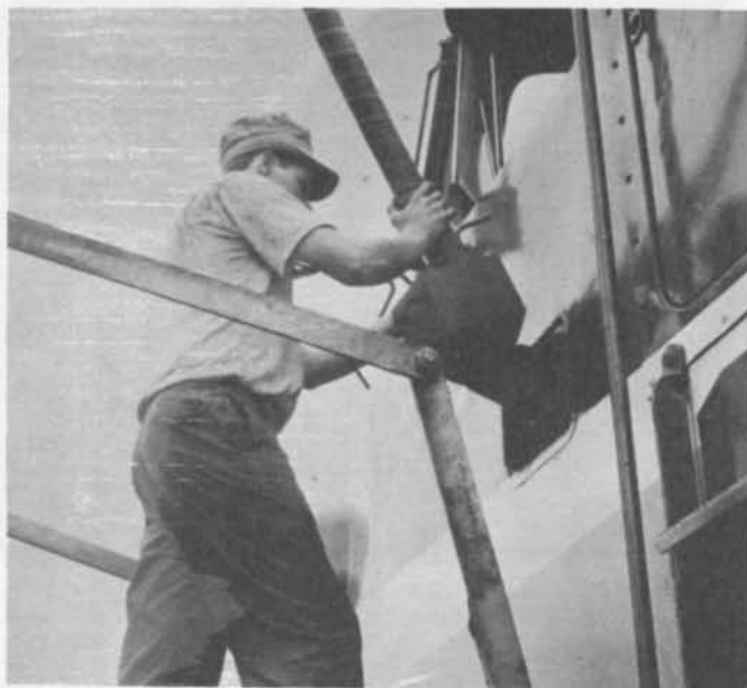
WHEEL SANDERS are also refilled on diesels' arrival for servicing, inspection and testing at the St. Paul Diesel shop. Locomotive pulls alongside sanding tower to receive a new load from a hostler helper.
