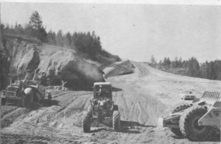
DUMPING FILL, earth mover, at left, dumps its load over section of fill area. Grader, in center, spreads and levels fill material into uniform layers. Fill in this area was 80 feet deep.
