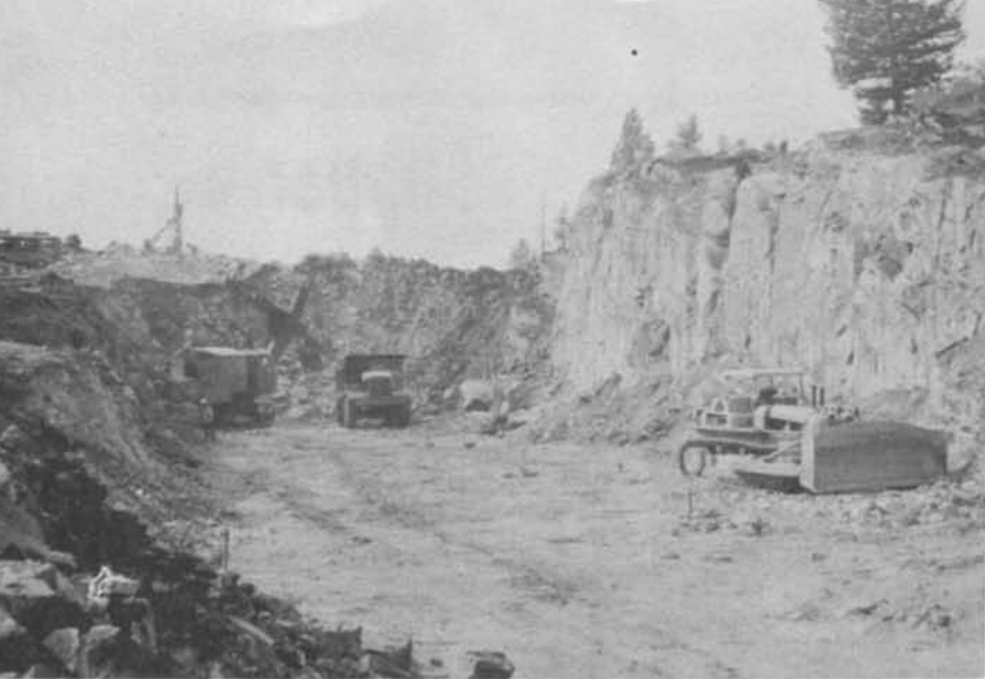
CARVING OUT the rock cut, a big power shovel loads truck with rock blasted from surrounding ridge. Tons of rocks were hauled to the swamp area and used as fill. Cover picture shows cut after completion.
