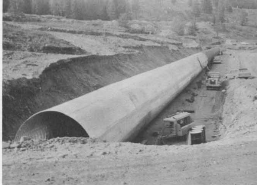
COMPLETED CULVERT, shown partly covered with butuminous coating (dark area), was entirely assembled on the site. 604 feet long, the culvert was covered with 115 feet of fill when the project ended.
