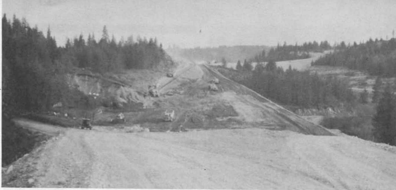
BIG FILL area, looking west of Granite, is seen crossing the swamp area at the upper right of picture. Earth movers, dozers, and trucks fill and grade stretch of road bed in foreground.
