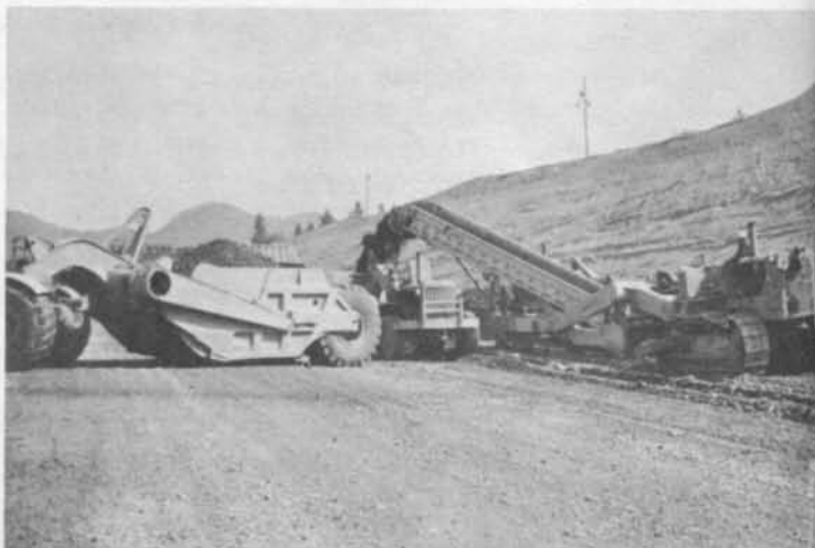
BIG CUT during construction stage shows belt loader in action. Crawler tractor, pulling loader, starts filling another large earth mover as loaded unit pulls away for the dump site.
