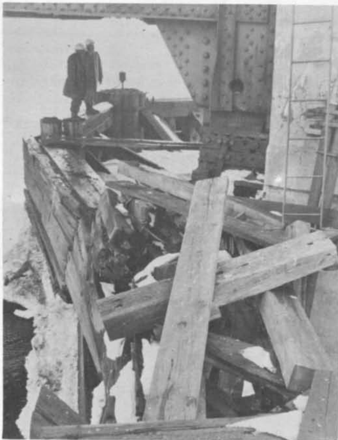
PIER 7, seen on Superior side of channel, was heavily damaged by blow of steamship when it veered off the bridge. Workmen, at top, inspect bridge after first closing was completed.
