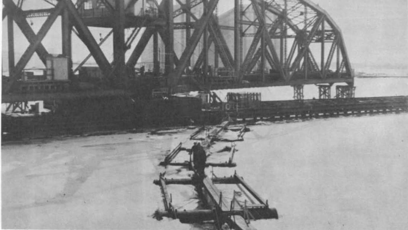
PONTOON BRIDGE, looking from the Duluth trestle, carried workers over frozen channel to work site on bridge. Temporary piling supporting damaged end is seen at upper right.
