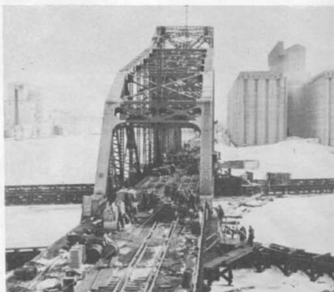
UNDAMAGED END of bridge seen from Duluth trestle, just after the bridge was first closed at end of repair work. Workmen, equipment and material cover bridge deck.
