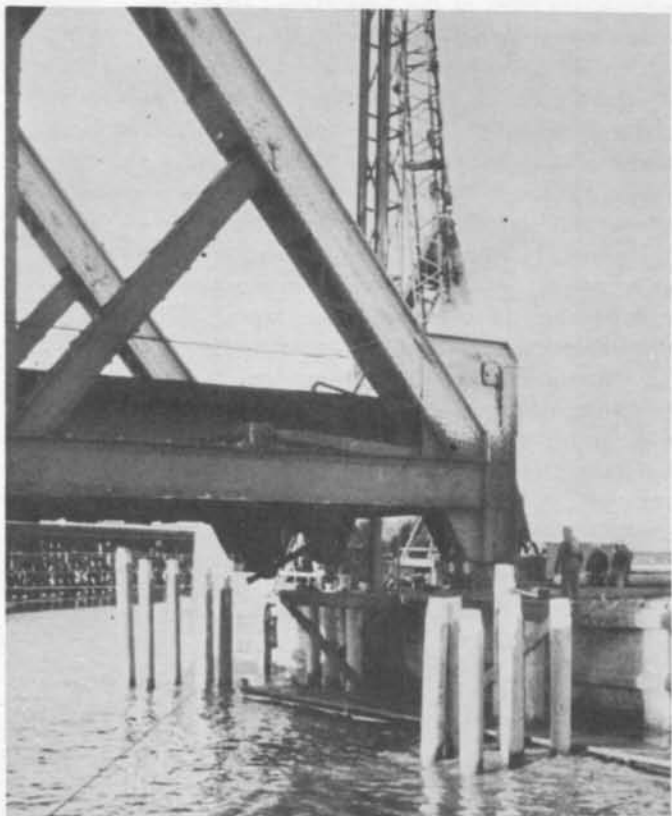
PIER 7, seen on Superior side of channel, was heavily damaged by blow of steamship when it veered off the bridge. Workmen, at top, inspect bridge after first closing was completed.
