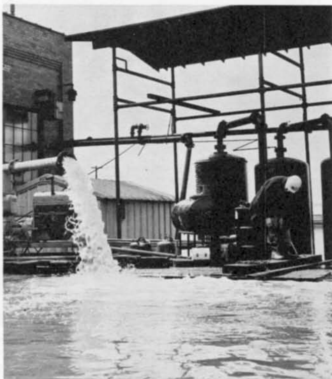
ISOLATED Water Service employee tends pump that ran continuously to prevent basement of Third Street power house from filling up.
