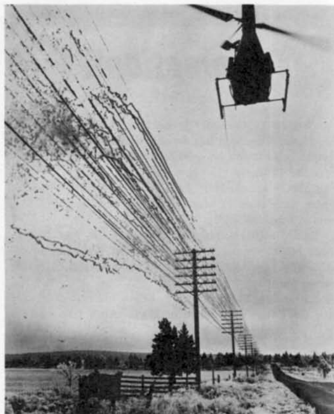
SNOW REMOVAL by helicopter is employed by the Northern Pacific when excessive attenuation threatens to disrupt service. Here a 'copter dislodges heavy accumulations of frost and snow from the company's lines between Spokane and Pasco, Wash.
