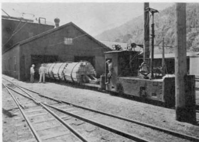
CROSS TIES are taken to the retort to be sterilized and treated with creosote preservative.
