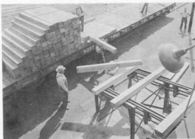
AIR-SEASONED TIES are unloaded and sent through NP's adzing, boring and incising mill.
