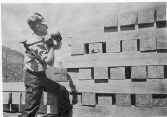
C-IRONS are driven into each cross tie to clinch wood fibers and prevent rail splitting.
