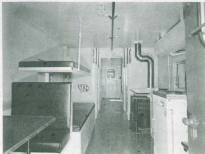
Inside View of Caboose Showing Stored Electric Marker Lamps, Stove, Table, Bunks, etc.
