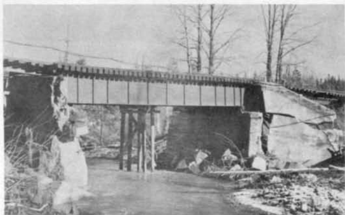
Abutments Heavily Damaged on Bridge 40
