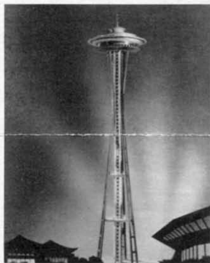
NEW SEATTLE LANDMARK —This 600-foot "Space Needle" observation tower, topped by the revolving "Top-of-the-Needle" restaurant, will be one of the feature attractions of the 1962 Seattle World's Fair. Two high-speed passenger elevators will carry visitors to the top, or to an intermediate platform, and the 220-seat restaurant. The latter will make a complete revolution each hour and will afford panoramic views of the lakes, mountains and salt water surrounding Seattle. The $2.5 million tower was designed by John Graham & Co., architects, Seattle and New York.
