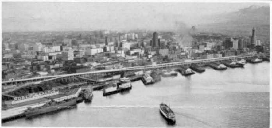
Seattle's new Alaskan Way Viaduct, spectacular two-level traffic overpass, stretching the length of the Puget Sound port's bustling waterfront, will be dedicated for use late in 1952—the Centennial Year of the Pacific Northwest's Queen City. (Seattle Times photo.)
