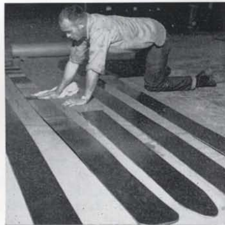
FROM HAFNIUM STRIPS made at Wah Chang, in Albany, Ore., rods are fashioned which control atomic reaction.
