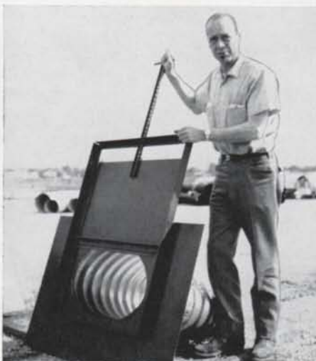
ADJUSTABLE STEEL GATES made at Missoula are like the one held above by C. G. Hesler, local manager for Roscoe.
