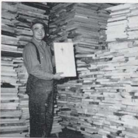
TAKING OUT KNOTS and trimming edges, Ernest L. Brookshier, above, gets clear lumber for use in his factory.
