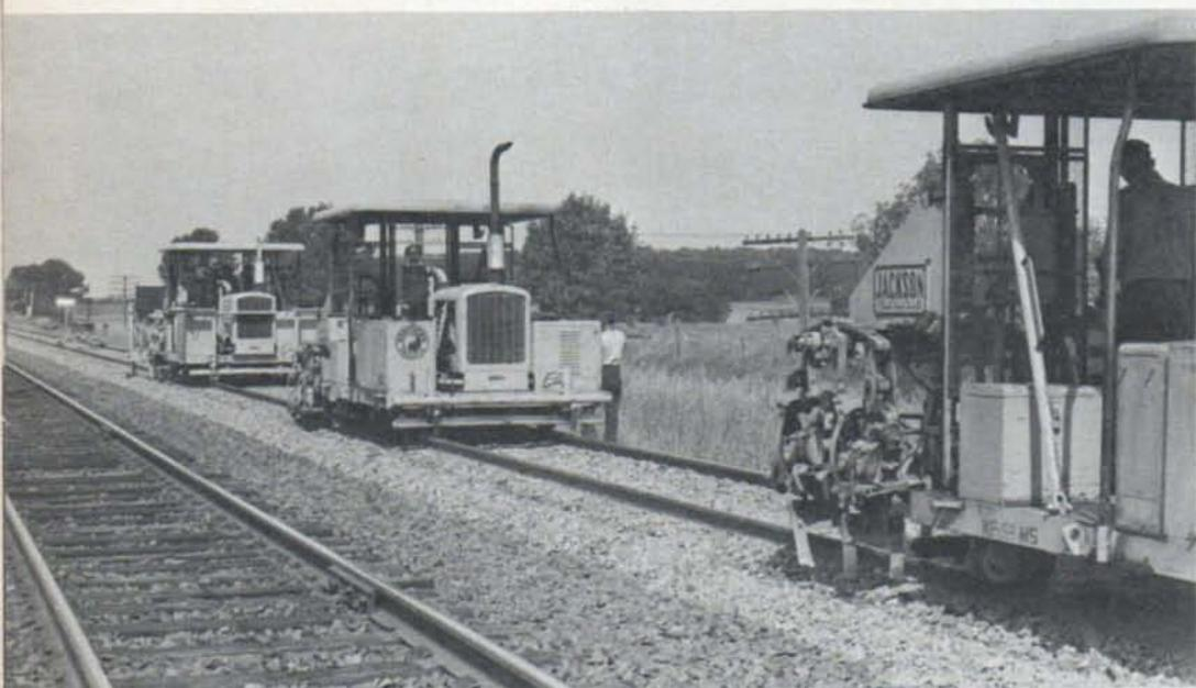
NORTHERN PACIFIC uses two conventional tampers (right) working in tandem with an automatic tamper at left. This technique increases production of surfacing gang.
