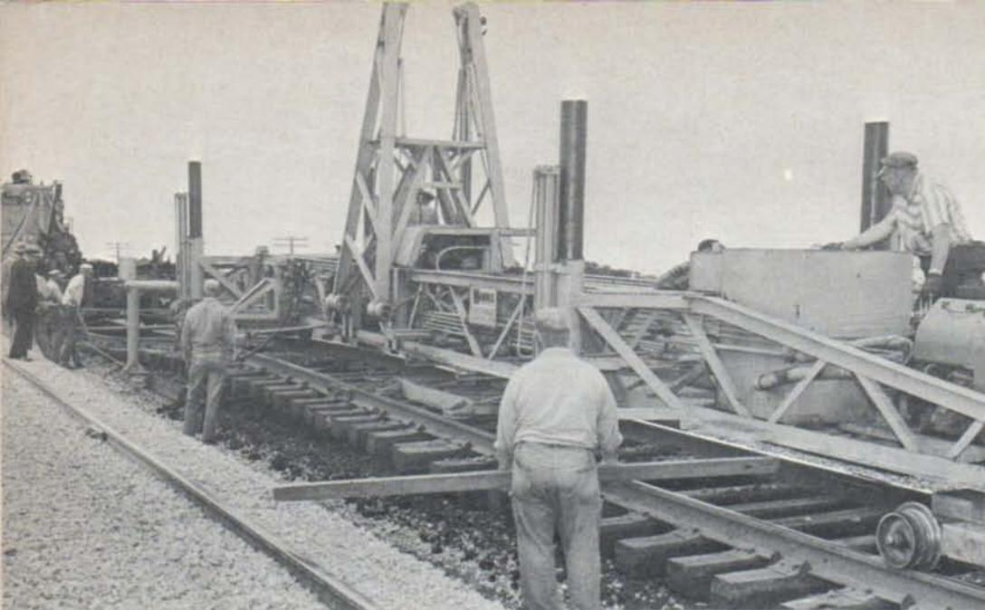
MODERN track equipment includes this multi-purpose machine that, when used with a ballast sled, picks up rails — ties and all — scoops out and levels old ballast, knocks out old ties that are to be replaced, lines the track and prepares roadbed for new ballast.
