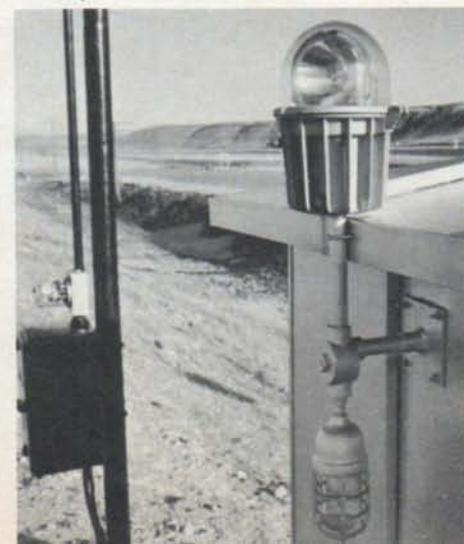
By the use of a reserve indication relay in series with the lamp filament, NP provides an approach aspect on the preceding signal when a lamp failure occurs. Power-off relays are provided to introduce approach lighting in the event the commercial power fails. The signals are then lighted from the reserve battery.
