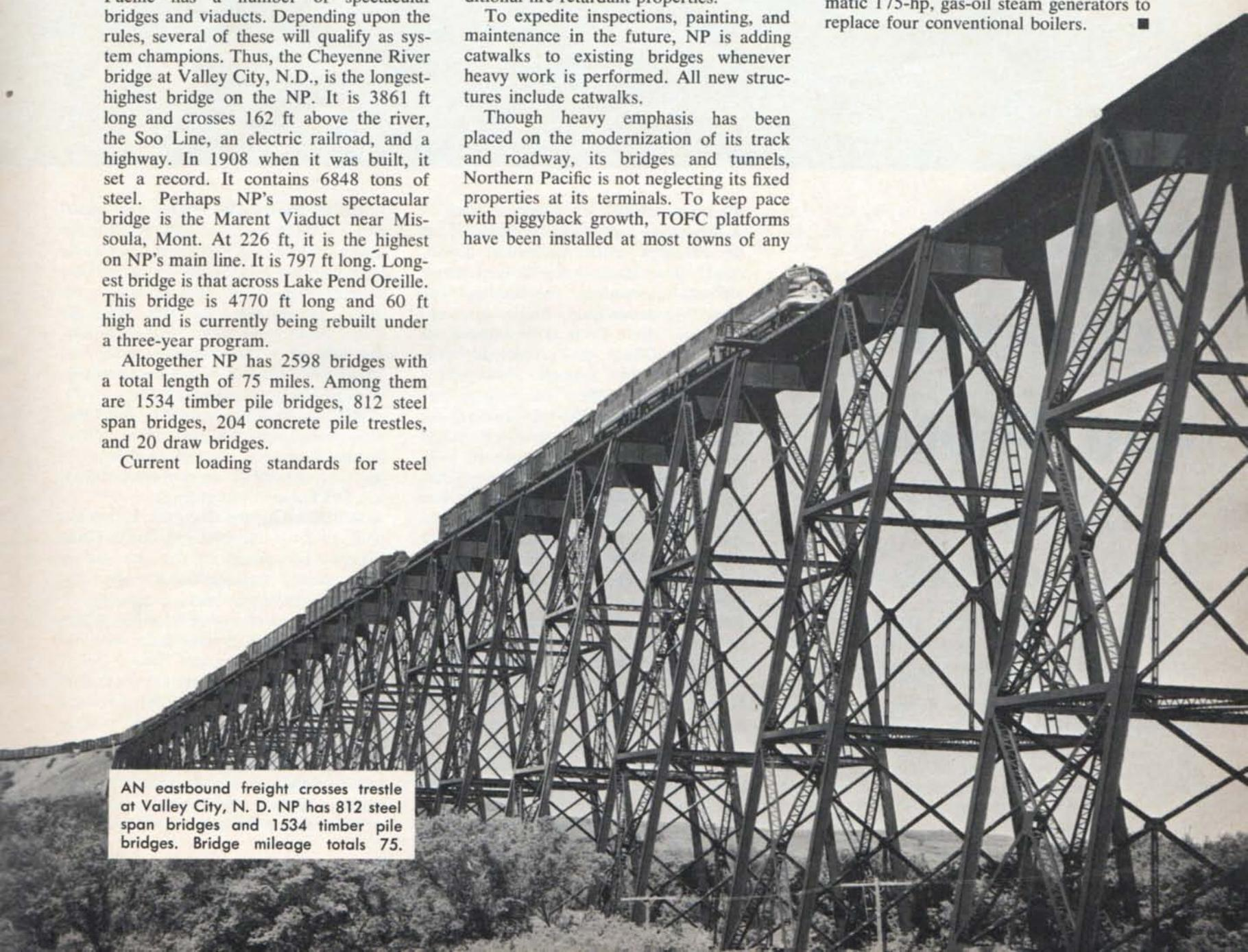
AN eastbound freight crosses trestle at Valley City, N. D. NP has 812 steel span bridges and 1534 timber pile bridges. Bridge mileage totals 75.
