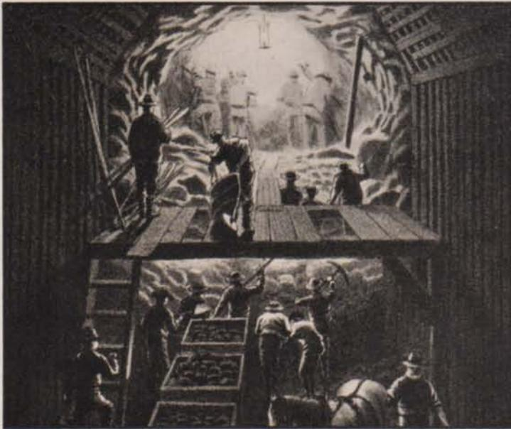
**A Two-mile Tunnel At Stampede Pass** in the Cascades was necessary to link Seattle directly with the east. The rough, tough Bennett brothers took on the job and on May 3, 1888, a final blast linked the two ends of the tunnel; the centers were within an inch of meeting perfectly.
