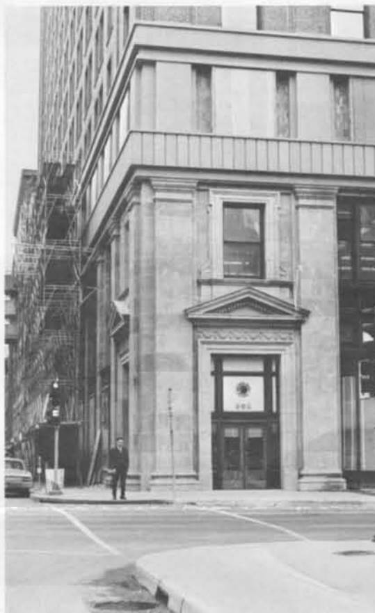
NEW EXTERIOR at the third floor level of the general office building in St. Paul awaits windows and panels of brown Duranodic 313 dark bronze. Later projects are planned which will match the exterior portion of the lower two floors to the New Third Floor exterior.
