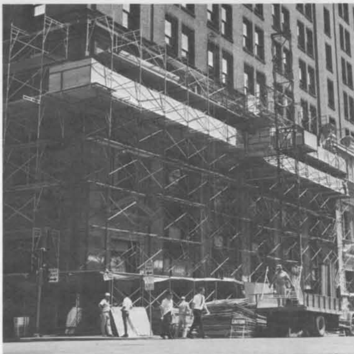
SCAFFOLDING , the steady drone of jackhammers, and dust were the steady diet for sight, sound and smell through much of the summer as workmen removed the huge sandstone ledge of the general office building at the third floor level.
