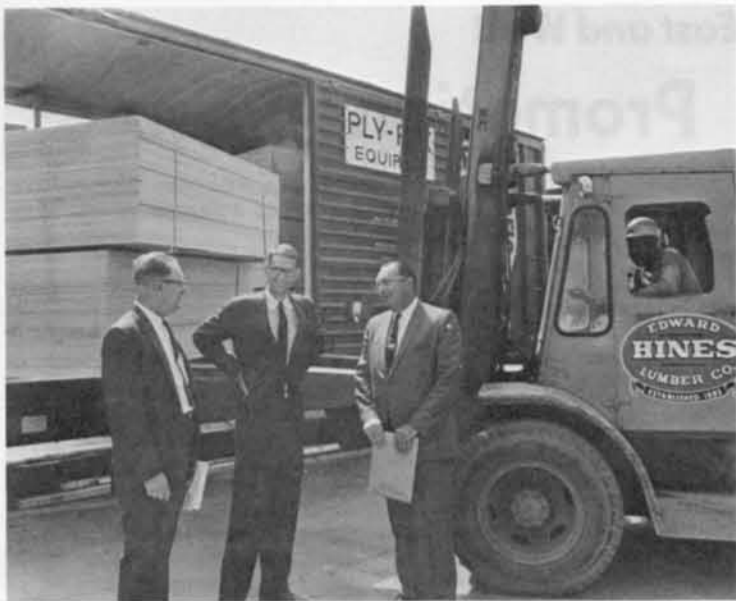
PLY-PAK EQUIPPED car speeded up loading and unloading. Left to right, Emmet J. Smith, director of transportation, Edward Hines Lumber Company; Edward Hines, vice president and general manager, Edward Hines Lumber Company; Harold J. Spence, assistant freight traffic manager, Northern Pacific Railway and Hines' fork lift operator, Gene Hollerway, all of Chicago, discuss new car.
