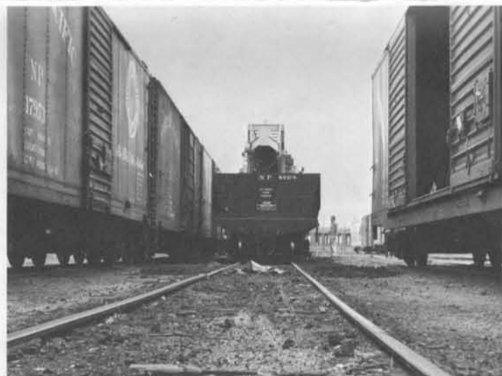
TRACK AREA before the yard cleaner passes through shows build-up of dirt and debris which completely covers ties and makes hazardous footing.
