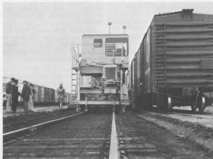
AFTER SEVERAL passes, the accumulation is finally cleared and loaded into airslide cars for removal to disposal area. Cleaning reveals need for tie replacement and other maintenance.
