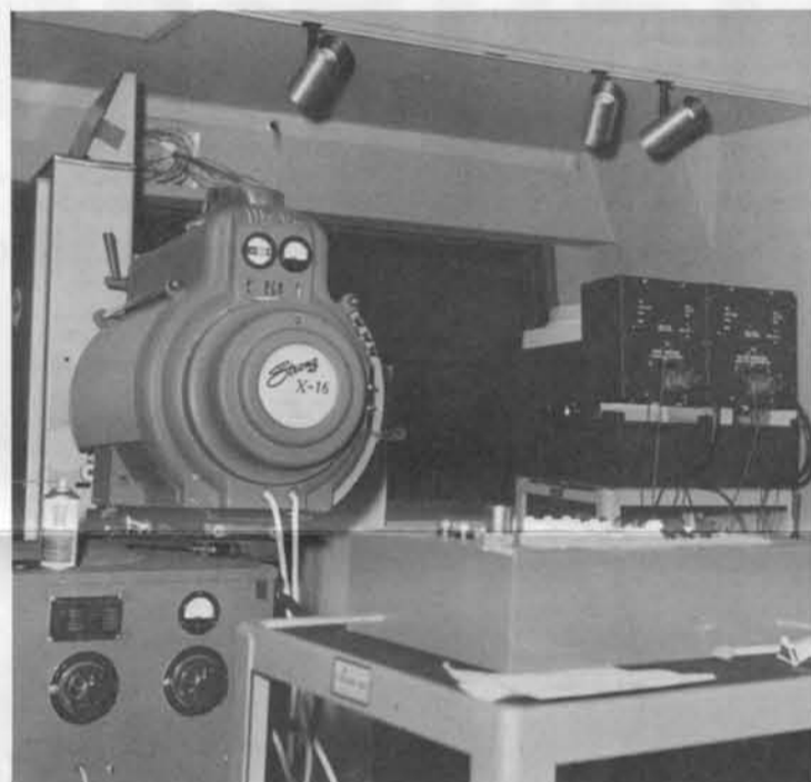
PROJECTOR FOR 35 millimeter movies, left, and twin carousel projectors, right, with high-intensity xenon light sources are part of the new visual presentation equipment in the new NP-GN auditorium in St. Paul.
