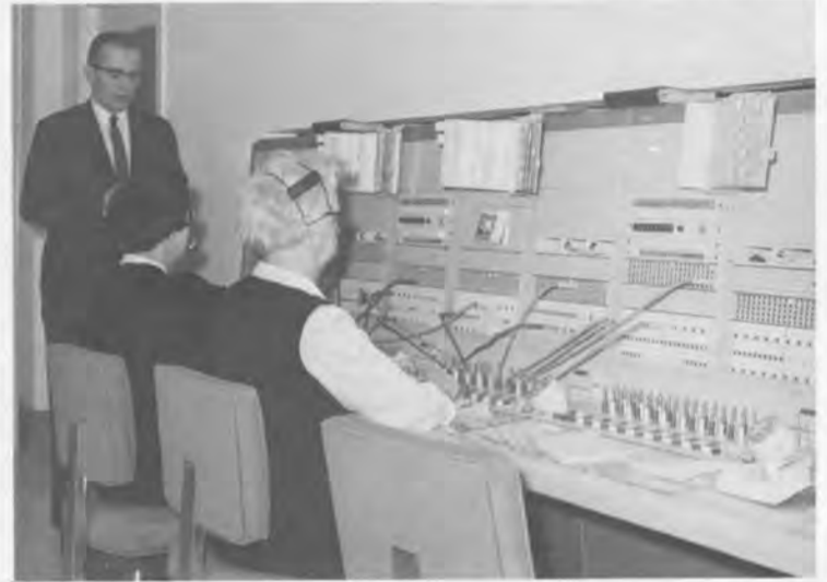
NEW 608 SWITCHBOARD in the St. Paul general office is checked out above by D. C. Hill, superintendent of communications. The board, with back-up equipment being inspected by Hill at left, is a 600 line unit which can be expanded to 700 lines. It handles incoming commercial calls, calls for inter-connection with the NP dial system, and outgoing commercial calls. The system was set up on second floor in February to make room for expansion of the NP dial facilities. Operators at the board are Mrs. Helen Cormier, left, and Ina Bergstrom.
