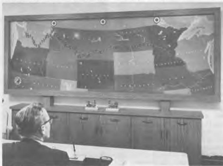
NP MICROWAVE CHECK-PANEL provides D. C. Hill, superintendent of communications, with immediate information on how the entire system is functioning.
