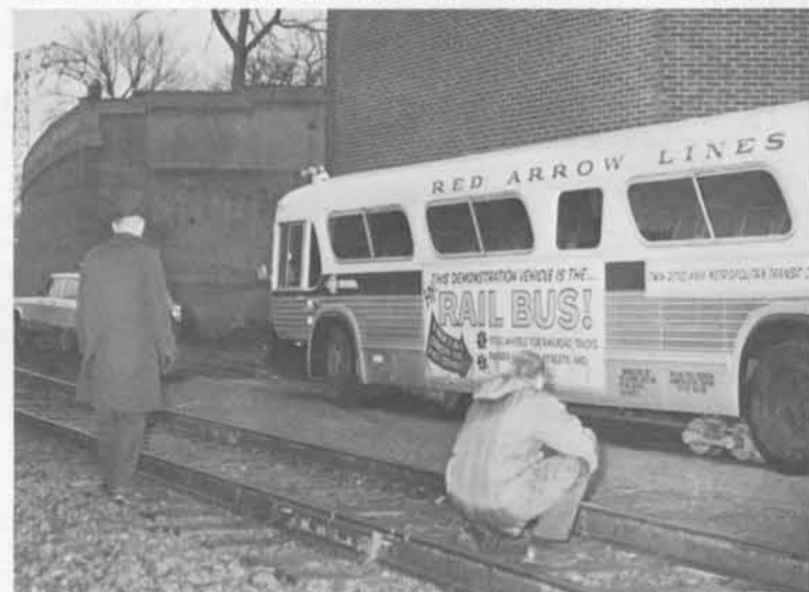
INTERCHANGE from road to railway operation is made by Fairmont's demonstration rail bus at a special loading area constructed by the Northern Pacific near the University of Minnesota power plant. Supervising the operation is J. G. Heimsjo, left, superintendent of the St. Paul division.
