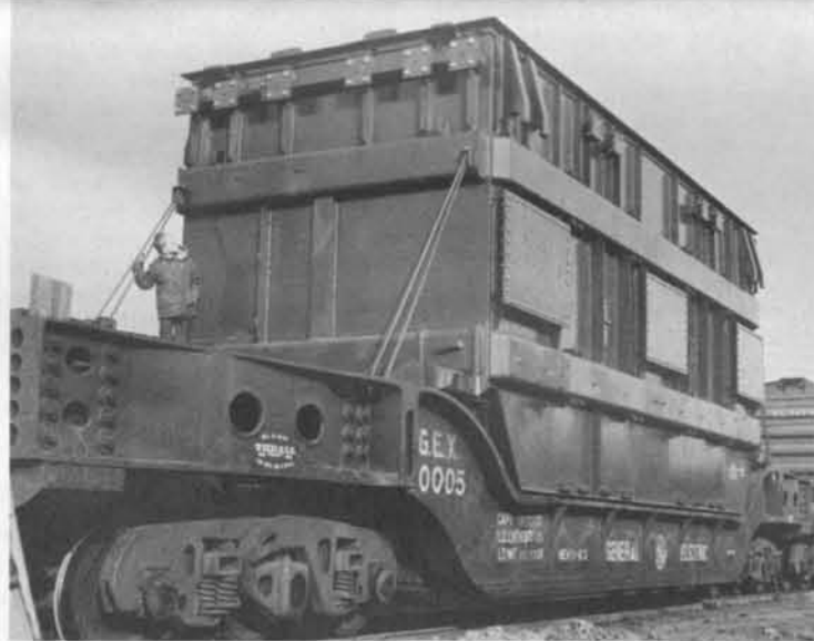
THIS 319-TON TRANSFORMER for Northern States Power Company's Alan S. King generating plant at Bayport, Minn., is one of the heaviest loads ever moved by the Northern Pacific. Gross weight with the car was 846,000 lbs. It was manufactured by General Electric Co. at its Pittsfield, Mass., plant, departed there on Nov. 7 and was delivered at Bayport on Nov. 20.
