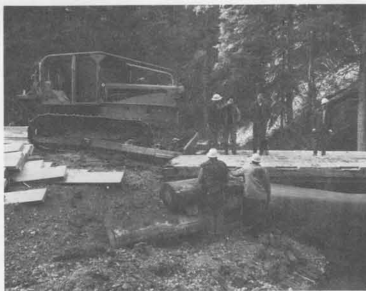
OLD BOXCARS NEVER DIE . . . and some from the Northern Pacific find new ways to carry loads. The timber division of the properties and industrial development department reports use of salvaged railroad car underframes for bridges on access roads to company timber lands in Montana. Timber contractors carry out the construction. This one, being built in the Jim Creek area of the Swan River tree farm near Missoula, is now completed and in use. Others are planned in the Swan River and Thompson River tree farm areas.
