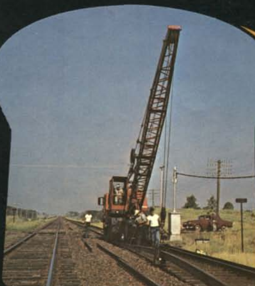
Tracklaying crews will relay 35 miles of main line with continuous welded rail.
