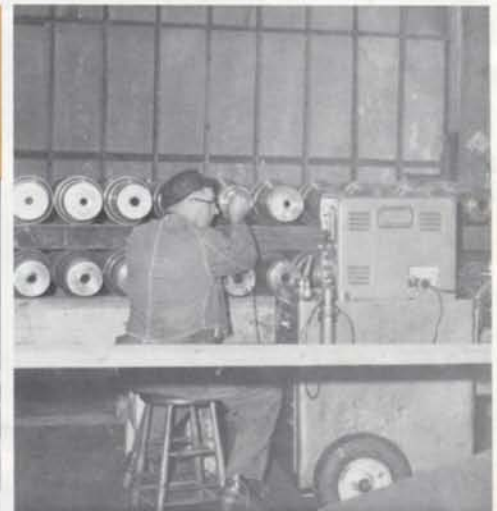
Harold Smith "looks" through a whole battery of axles with the reflectoscope.
