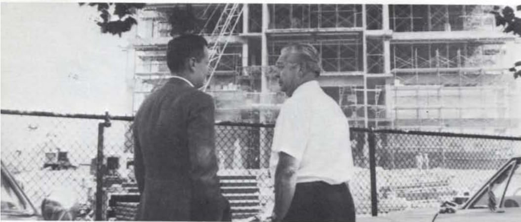
Harold Johnson, right, explains to Larry Kiser that Morrison-Knudsen Company's new Boise headquarters will provide underground parking for employee's cars.
