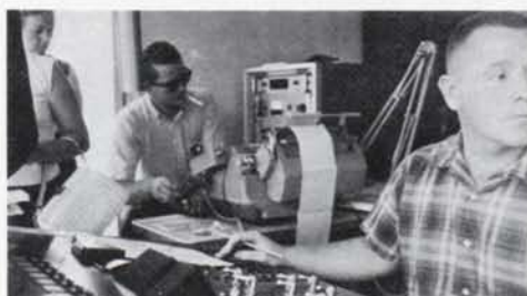
Pete Day (in dark glasses) operates the business end of the weigh-in-motion scale. Without stopping, each car is weighed and that information is printed on a ticket. At the control panel is Jim Bisette.
