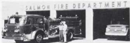
Salmon Fire Station and Diesel Truck.
