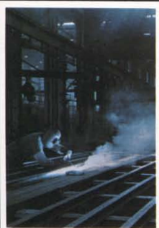
Underframe of a new Ply-Pak car takes shape in blue light of a welder's arc at the Brainerd shops.
