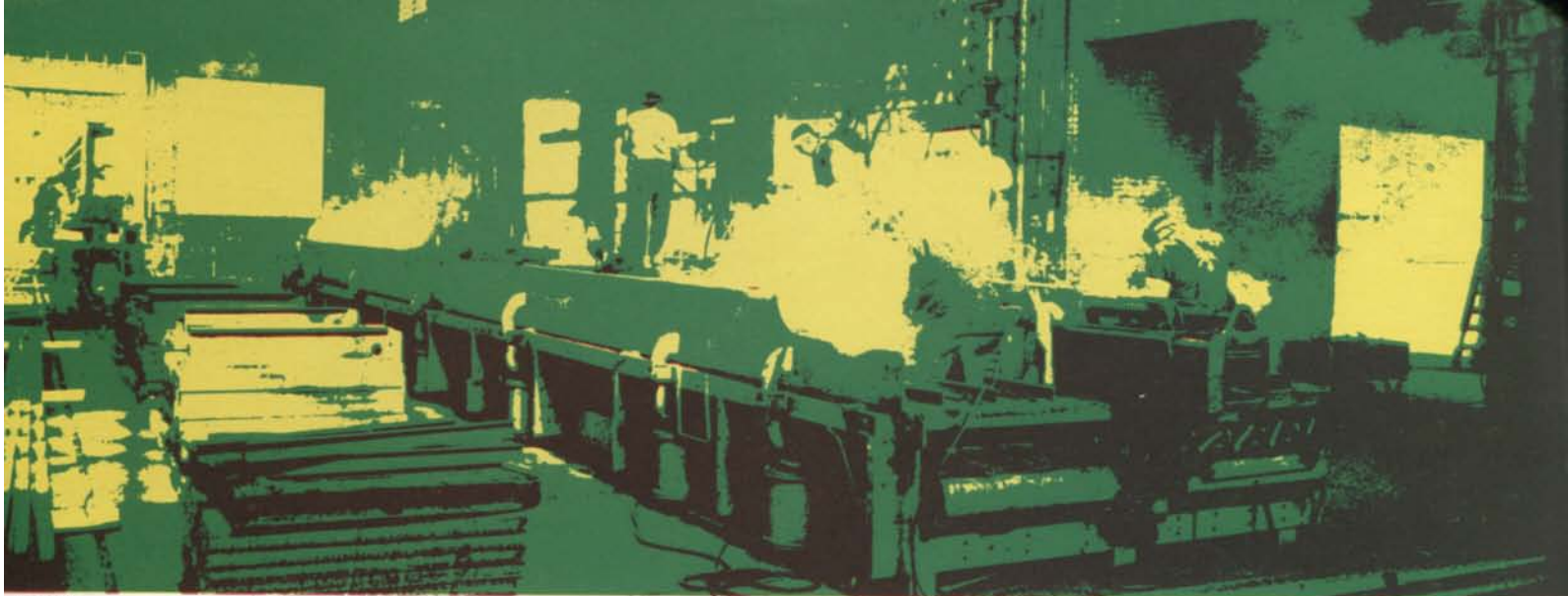
Welders swarm over underframe in laydown jig.
