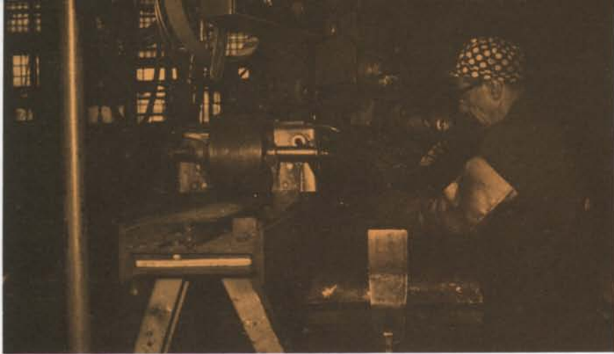
Lawrence Bourassa uses submerged-arc welding machine to join end sections.
