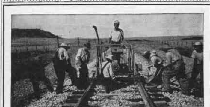
Roadbed improvement is a continuing program on the Northern Pacific
