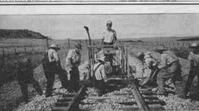
Roadbed improvement is a continuing program on the Northern Pacific
