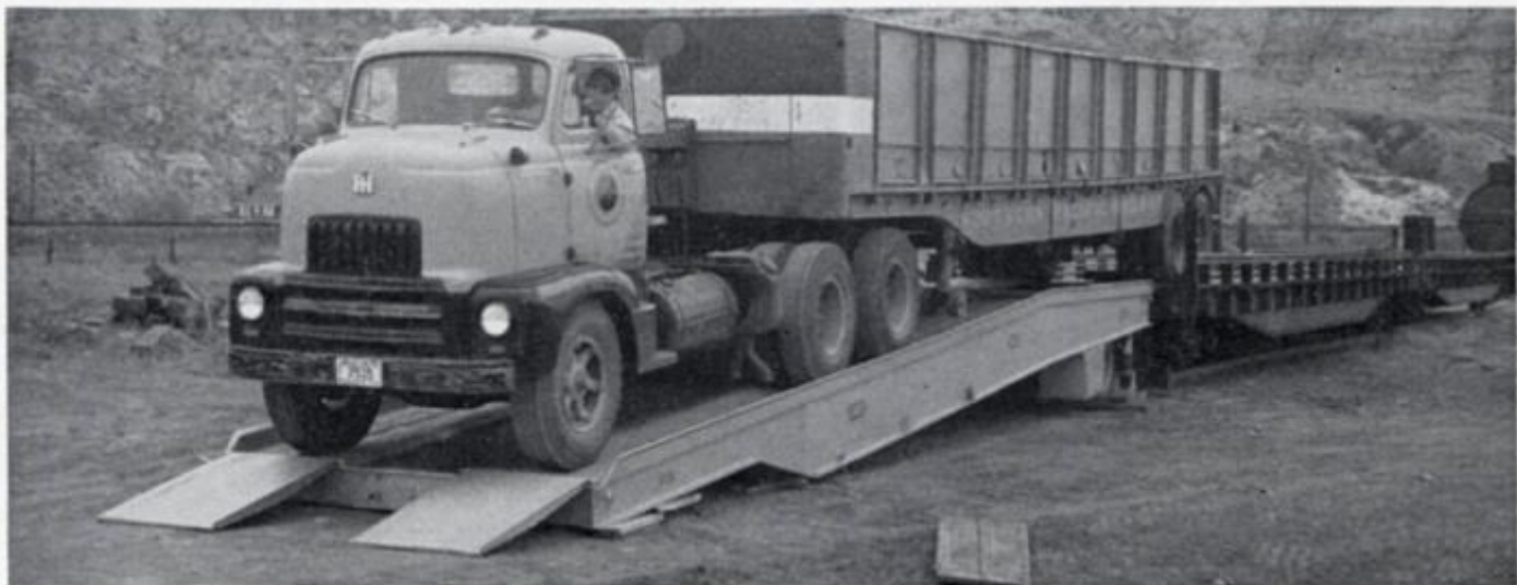
A PIGGYBACK TRAILER carrying reinforcing steel for a new bridge at Medora, in western North Dakota, was moved with a portable ramp from a flatcar on the rail-road to the site of the construction. The ramp was used similarly at South Heart, N.D.
