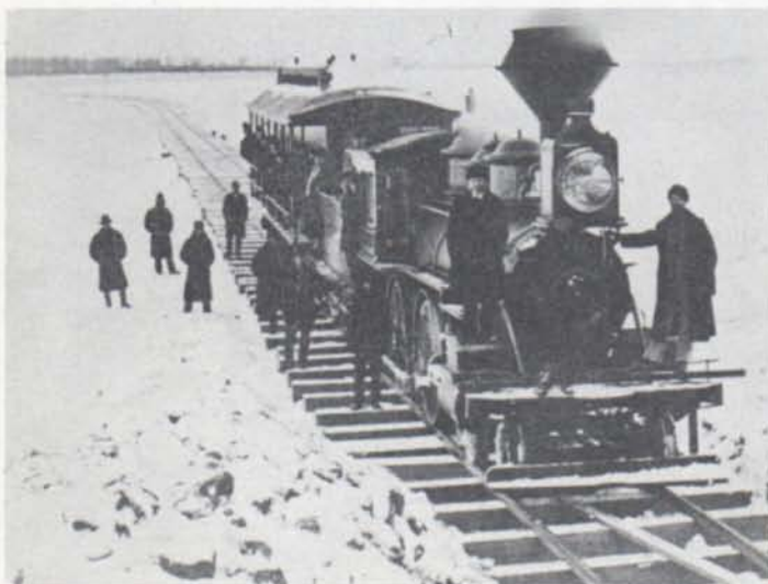
RAILS ON ICE allowed Northern Pacific trains to cross Missouri River from Bismarck to Mandan during winters of 1879-82.
