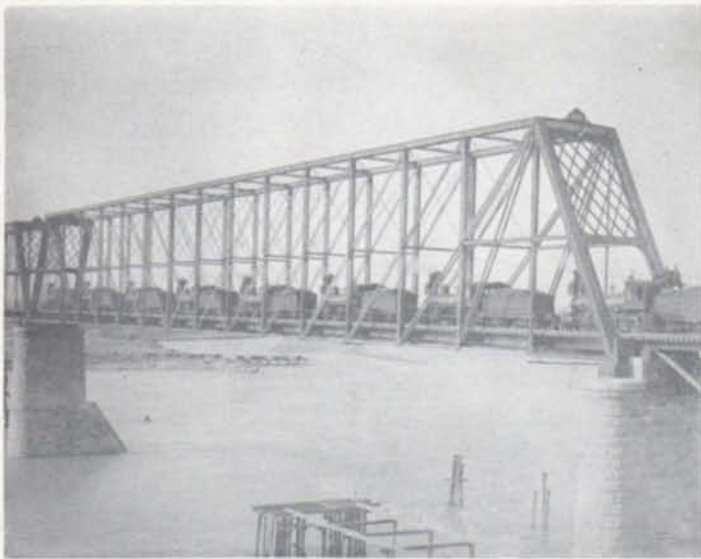
TESTING NEW BRIDGE--a fleet of NP locomotives are sent on test run over Bismarck Bridge on Missouri River on Oct. 23, 1882.
