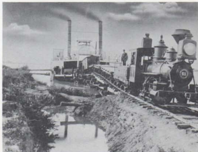
FERRY BOATS carried NP trains back and forth over Missouri River in summer. Bismarck Bridge was completed in 1882.
