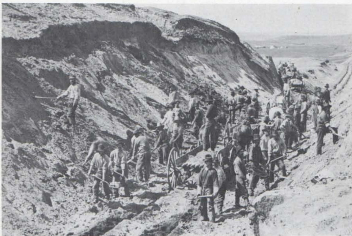
NP grading crew constructing railroad right-of-way in Dakota Territory, 1879.
