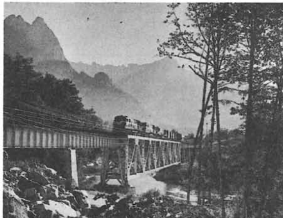
Great Northern's last major line change before merger was multi-million improvement project in Cascades, begun in 1961 and completed in 1968. Eastbound freight is pictured on new bridge across Skykomish River.
