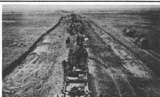
Scenes from record-breaking year of 1887 show track being laid across virgin prairie in Dakota Territory, and St. Paul, Minneapolis & Manitoba work train with unusual tri-level dormitory cars.
