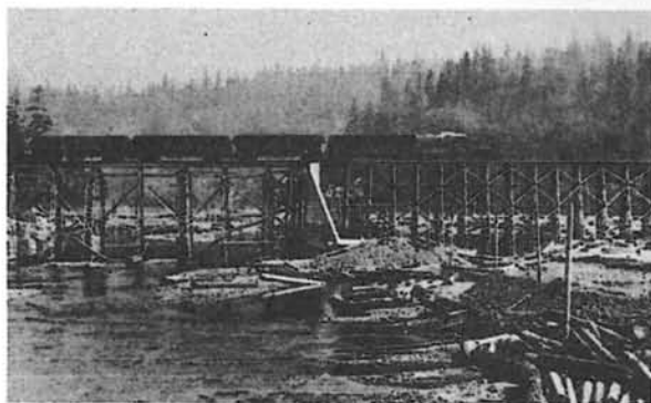
Passenger and freight runs along segments of the SP&S North Bank line began shortly after the start of construction in 1905. In this photo a temporary trestle spans Hamilton Creek near North Bonneville.
